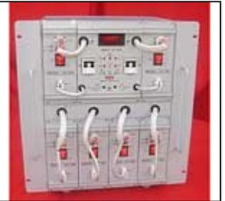
MODEL DY 6350 is a Modular Power System, which uses 6 nos. Hot-Pluggable DY 350 Rectifier Modules of 350Watts.
